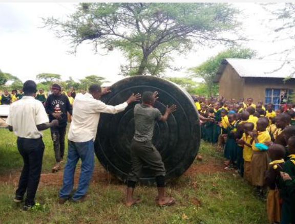
The community helped install the tanks for their local schools
